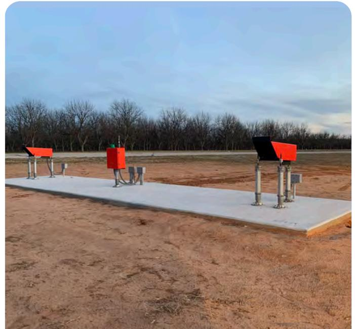
*The Series 3 PAPI is Intertek certified to FAA AC 150/5345-28H. Patented LED technology provides the highest intensity, sharpest red/white transition line, and lowest power consumption.*
