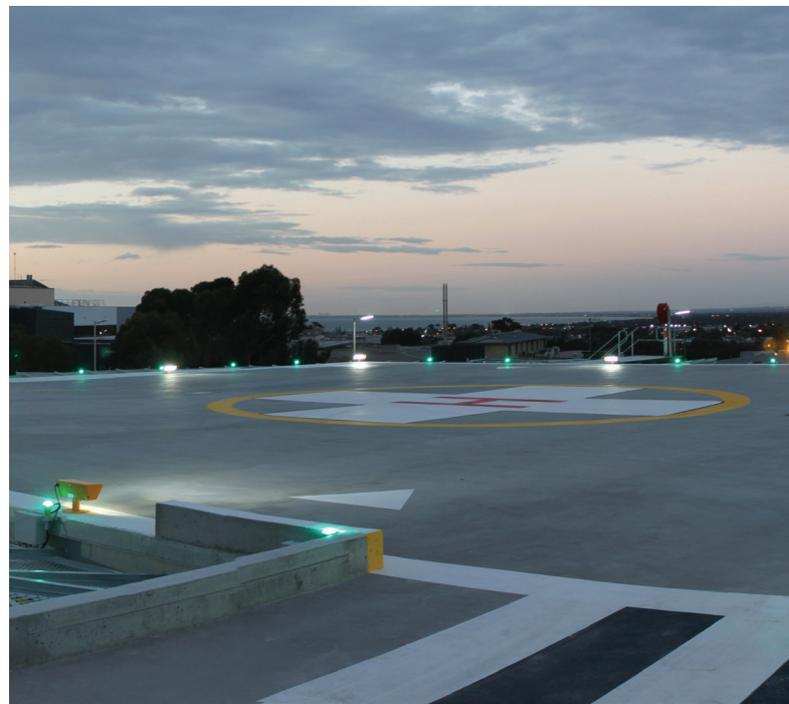
“The flood light demonstration illustrated the very neat tilt-adjustment feature that allows fine-tuning of the luminaire to provide the best light-spread across the heli deck without dazzling pilots upon approach,” he added. “Since the luminaire is LED driven – with a life of up to 100,000 hours – our client will never need to worry about changing a light globe, ensuring this reliable, low-maintenance fixture has a low cost of ownership over its lifetime,” Mr Simpson said.
